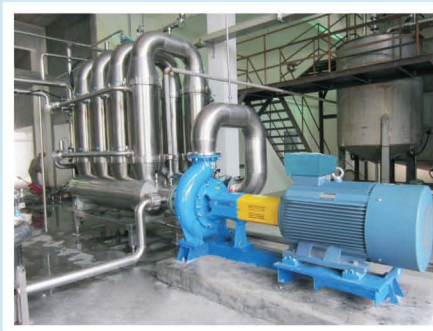
Ceramic membrane plant on site
